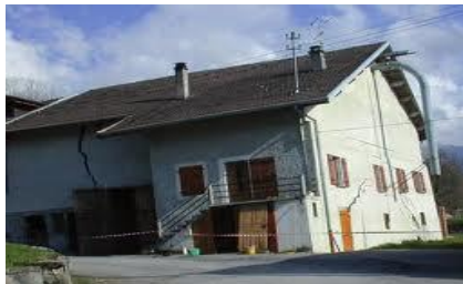
Subsidence on clay soils, 2011
